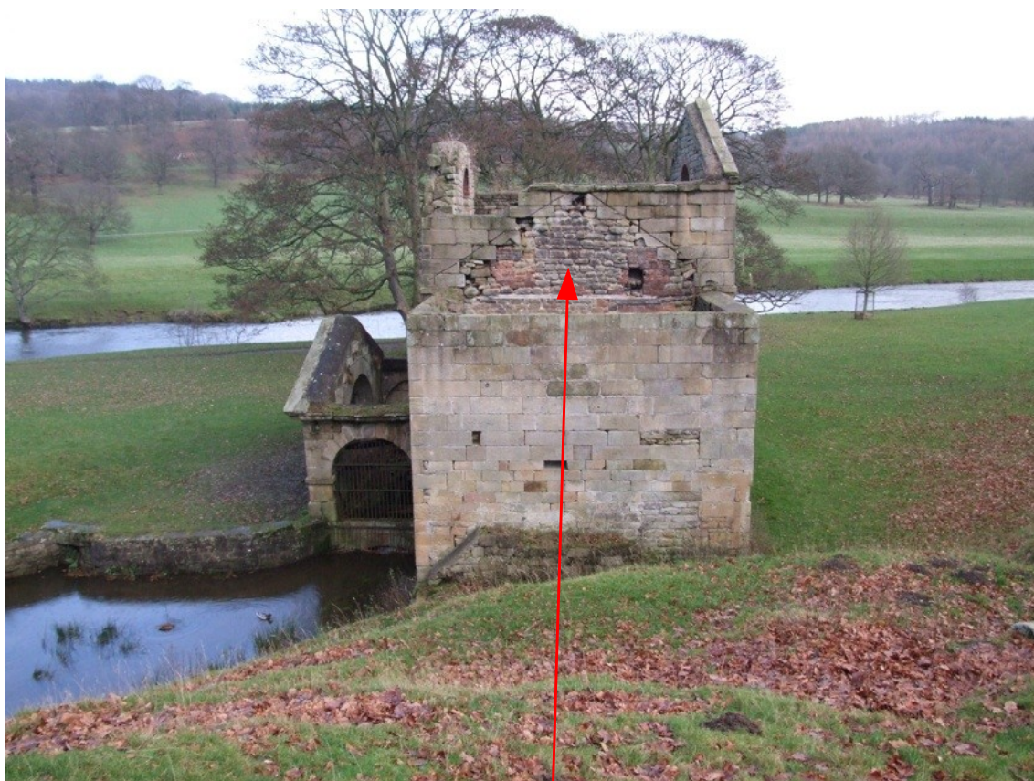
Photo 4: The west side - note rough masonry of internal wall at apex
