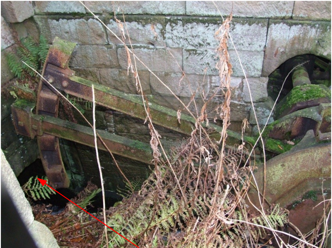
Photo 11: Water exit tunnel and remains of mill wheel
