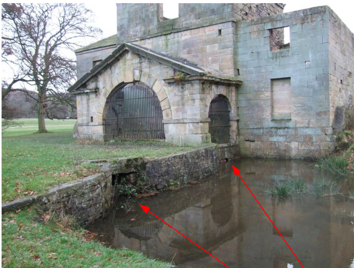
Photo 9: The wheel house, end of the millpond, bypass sluice and pond weir
