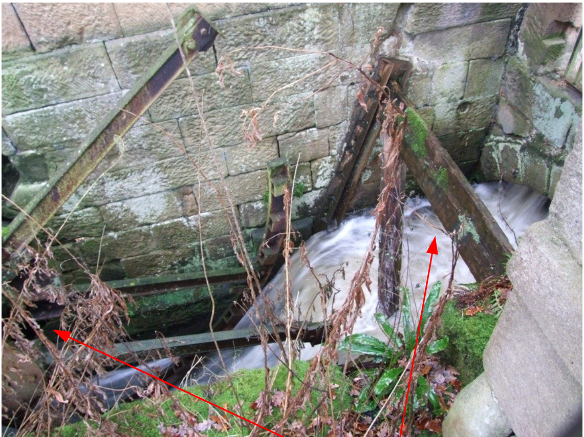
Photo 12: Remains of the mill wheel and control gate
